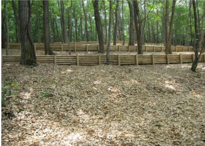
*FIG. 2.5: Application of wood chips as a countermeasure to reduce the air dose rate in a forest (Image: Fukushima Prefecture).*
